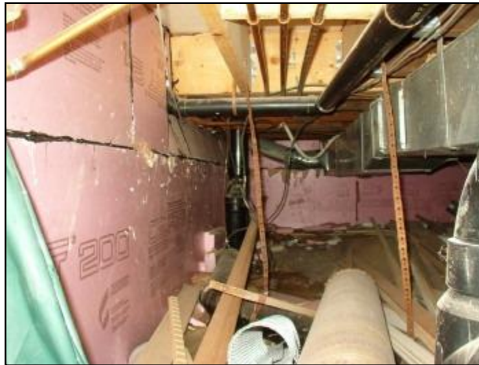
12. Exposed combustible insulation
