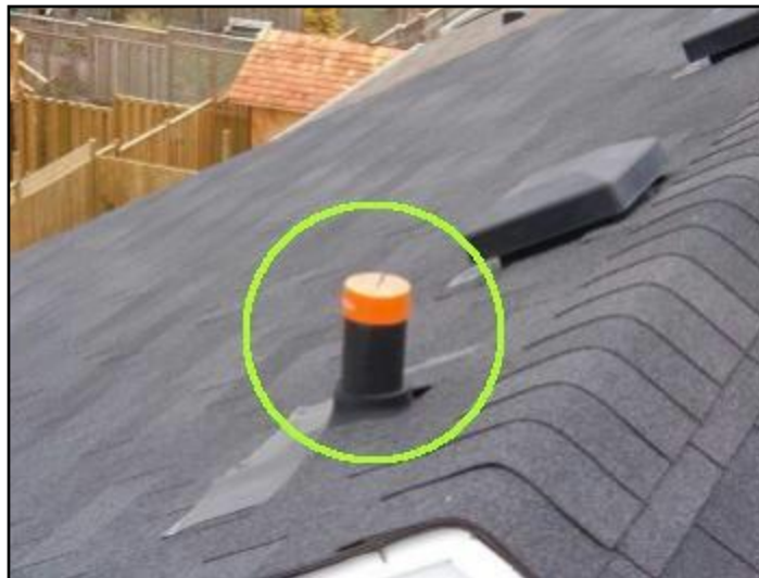
15. Plumbing stack is capped
