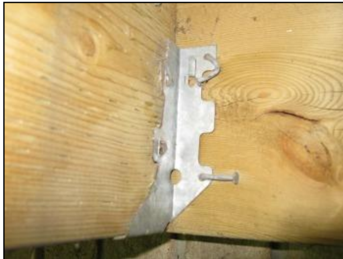
4. Poor end bearing, joist hanger connections
