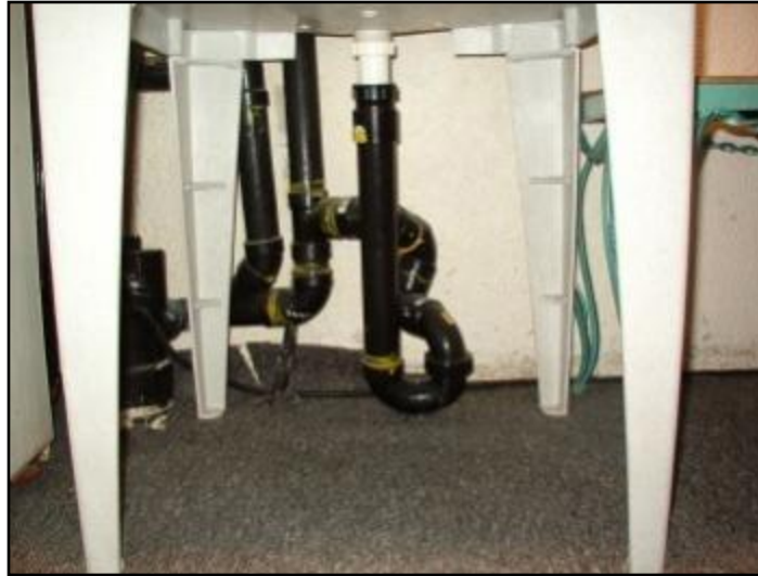
14. Poor trap arrangement
