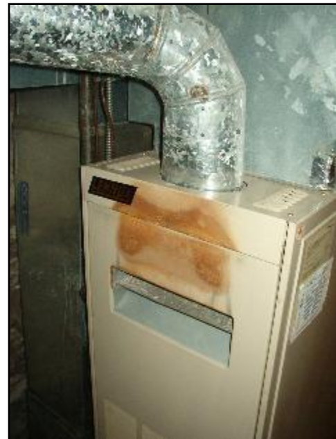
10. Draft hood spillage or backdraft
