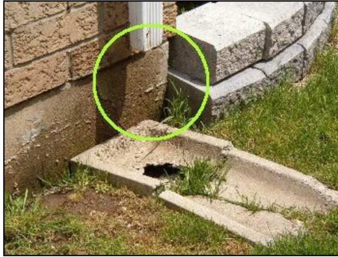
3. Downspouts discharge too close to building
