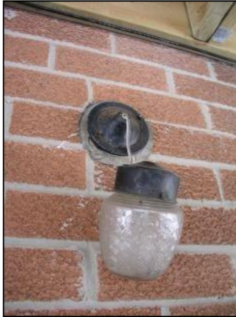
8. Light fixture is not well secured
