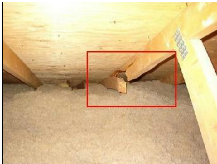
6. Top chord of truss is split
