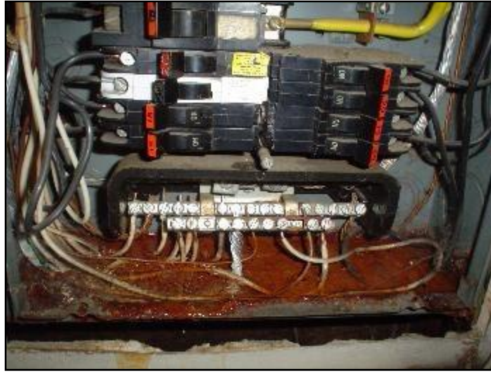
7. Water and rust in bottom of panel
