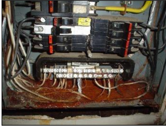
7. Water and rust in bottom of panel
