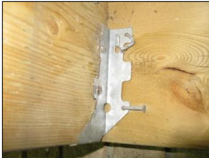
4. Poor end bearing, joist hanger connections
