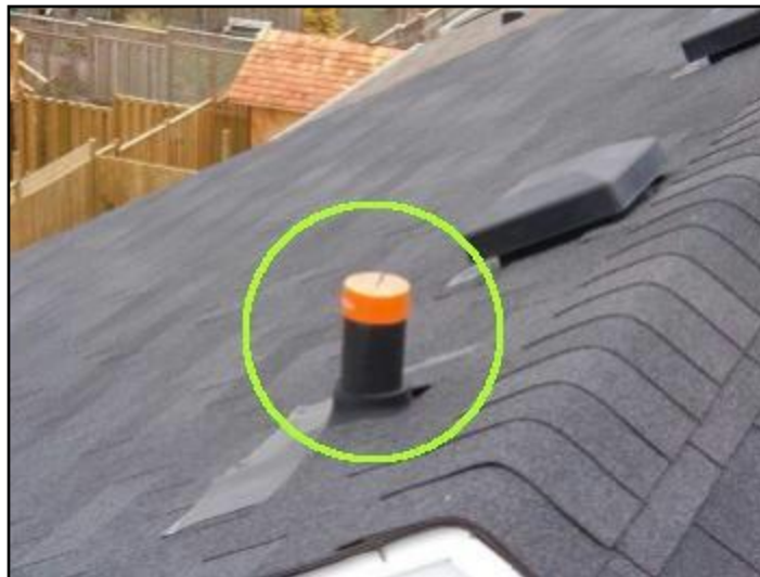
15. Plumbing stack is capped
