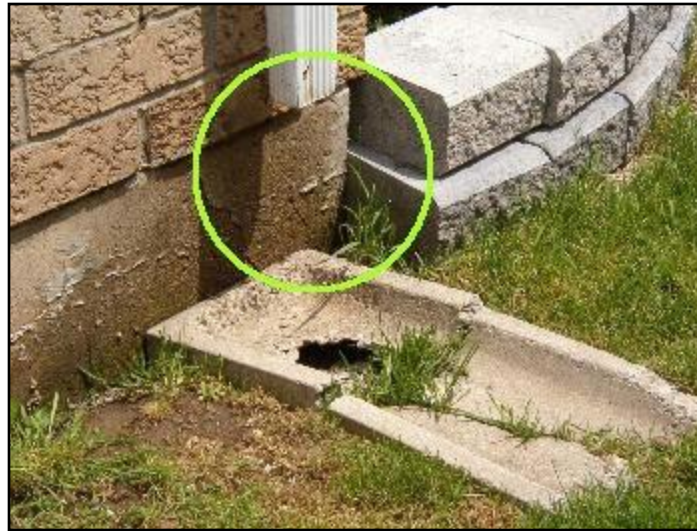
3. Downspouts discharge too close to building
