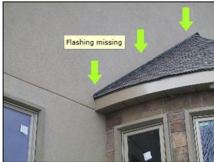
1. No kickout flashing at roof/sidewall junction
