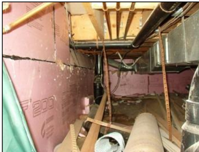
12. Exposed combustible insulation
