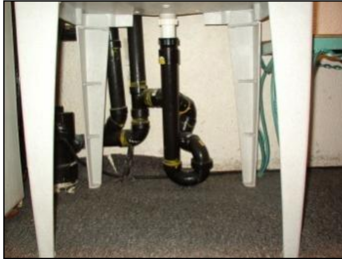
14. Poor trap arrangement
