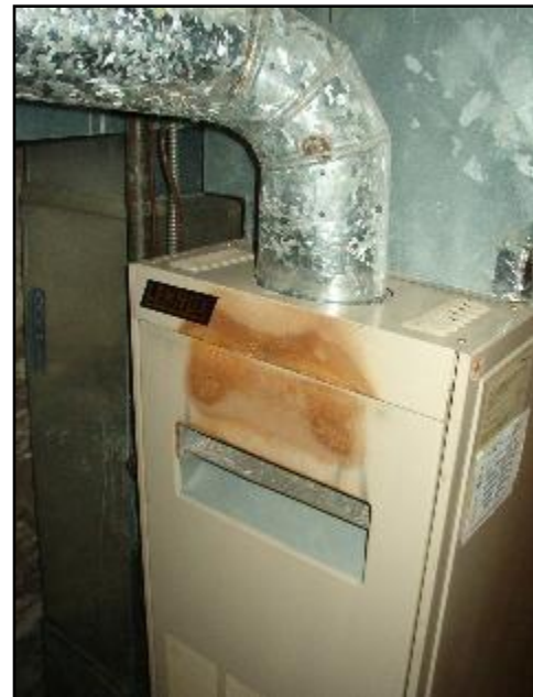
10. Draft hood spillage or backdraft
